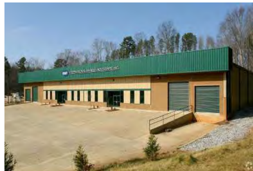
Our Distribution Center
